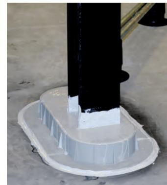
*Even large penetrations such as H-beams can be sealed using the right combination of E-Curb straights and curves.*
