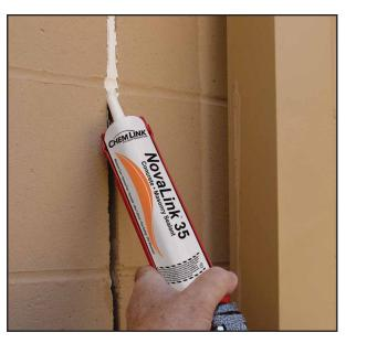
**NovaLink 35™** is a multipurpose polyether construction sealant specially formulated for application in damp, dry, or cold job site conditions. **NovaLink 35** is UV resistant and will not suntan. **NovaLink 35** is SWR Institute validated for +/-35% joint movement. **Novalink 35** is designed for use with many building materials including glass, concrete, metal and most roofing materials.
