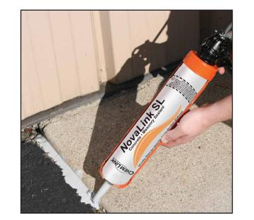
NovaLink SL™ is a self-leveling polyether construction sealant specially formulated for application in damp or dry horizontal concrete expansion joints. It is highly UV resistant and will not suntan. NovaLink SL will not outgas or bubble when applied to damp concrete. NovaLink SL is safe to use on EPS foam insulation.
