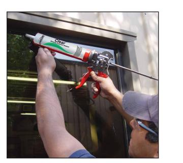
Clear™ is a multipurpose polyether based, high-performance sealant that can be used to seal a wide range of construction materials. Clear forms a translucent, elastic, waterproof seal to most painted metal, anodized aluminum, glass, vinyl, wood, masonry, polystyrene and many engineered plastics.
