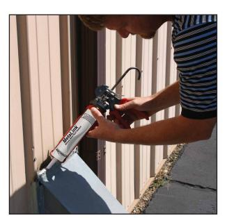
MetaLink™ is a multipurpose neutral cure silicone sealant specially formulated for application in damp, dry or cold job site conditions. MetaLink is UV resistant and will not suntan. MetaLink is designed for use with many building materials including glass, concrete, Kynar 500 PVDF coated metal and most roofing materials. With 50% joint movement, MetaLink is highly elastic, so it resists cracking, even through extreme weather cycles.
